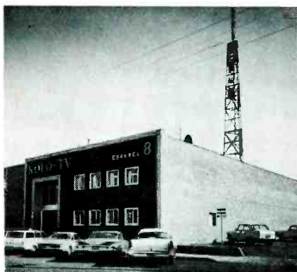
Reno terminal of the microwave system.
